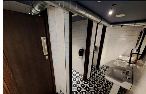
Washroom plumbing and fitout
