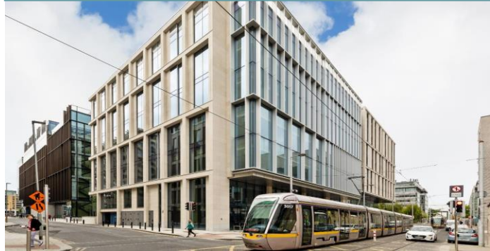
Building 3, Spencer Place, Dublin 1
